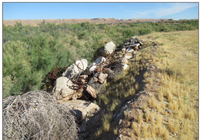
Virgin River, Bunkerville East, Parcel 2-E; Top of construction debris/dirt berm along edge of the tamarisk forest
